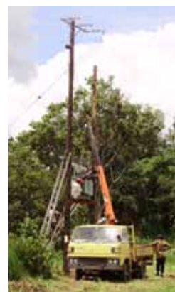
Above: The full extent of the Zambezi Rapids hydro-electric scheme as seen from the air. Right: An implementation team installs a distribution transformer that will power up a mobile phone tower.
